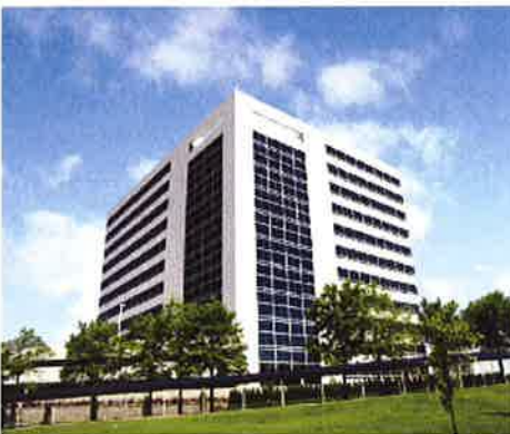
Tower One at 1250 Waters Place - Bronx, NY
