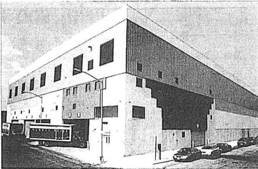
Photo courtesy of Simone Development
