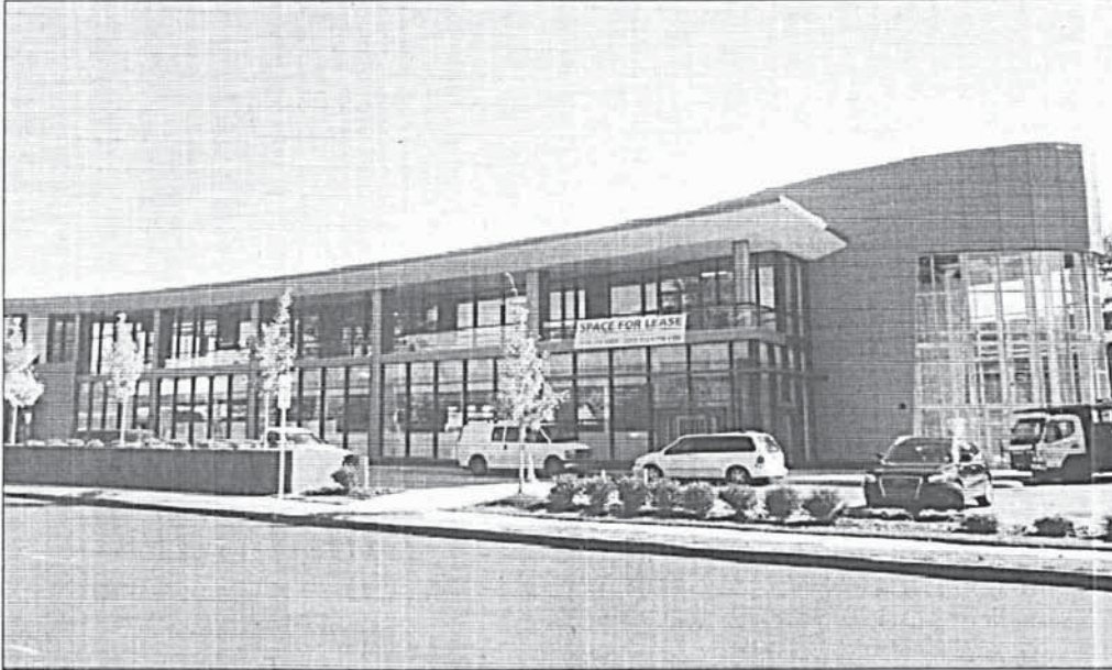
The building at 644 West Putnam Ave. welcomes CVS as its first tenant.
